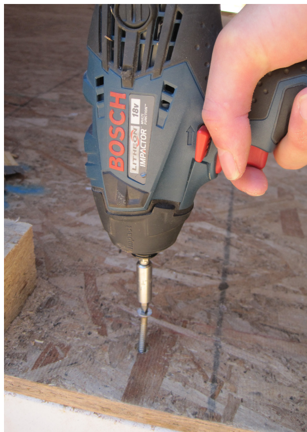
Drilling holes and installing field nails.
