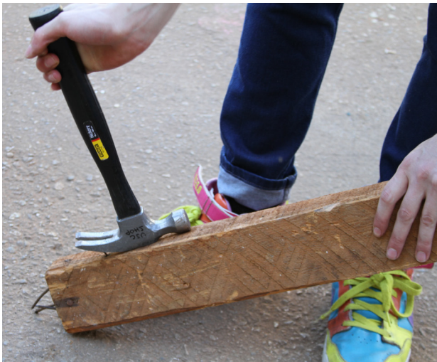
Pulling nails from reclaimed lumber.
